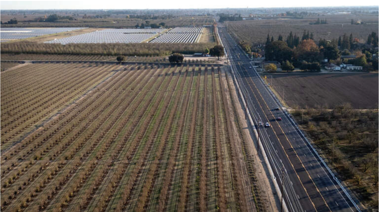
Looking south from the newly widened McHenry Avenue west of Riverbank, Calif., Saturday, Dec. 9, 2023. Andy Alfaro aalfaro@modbee.com
