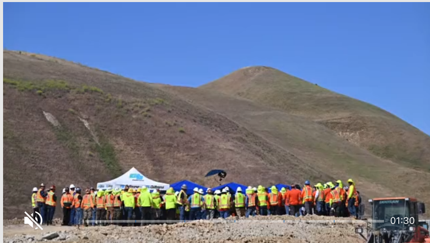
See giant solar project under construction near Patterson
